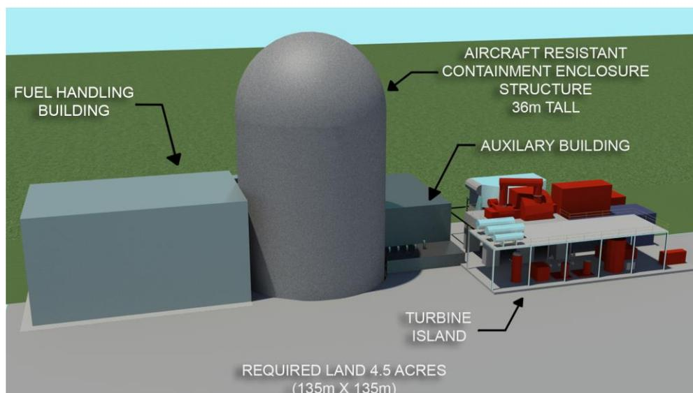
A typical SMR-160 uses cooling water from a local natural source such as a lake, river or ocean to condense its exhaust steam. However, it can also be deployed in water-challenged regions by using air as the condensing medium. Note that a SMR-160 in an arid region will typically produce about 3% less power and require about one more acre of land.
